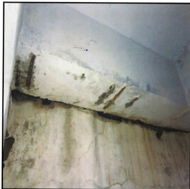
Steel Exposed at Beam and Leakage at Construction Joint
