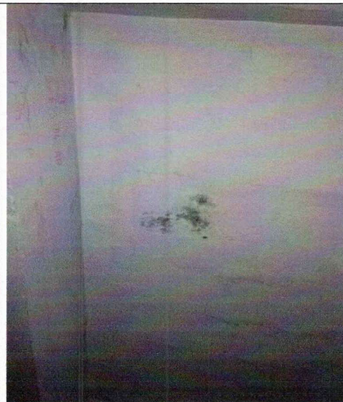
Dampness marks on slabs.
