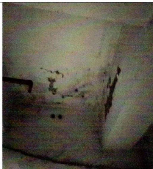
Leakages/Dampness marks on slab, peelings of paint.
