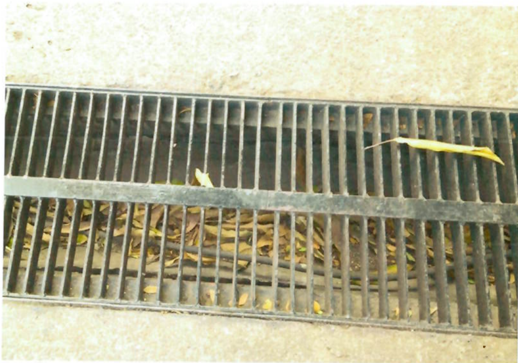
Fig. 14 Drains filled with dry leaves
