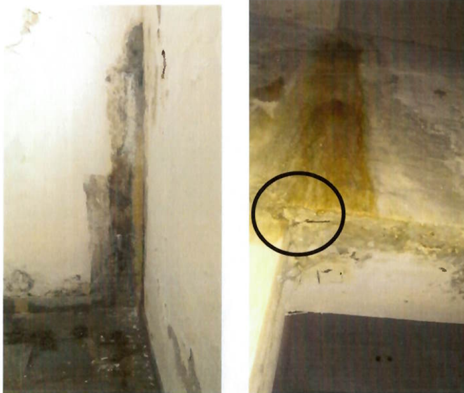
Fig. 5 Water seepage at wall and beam column junction.
