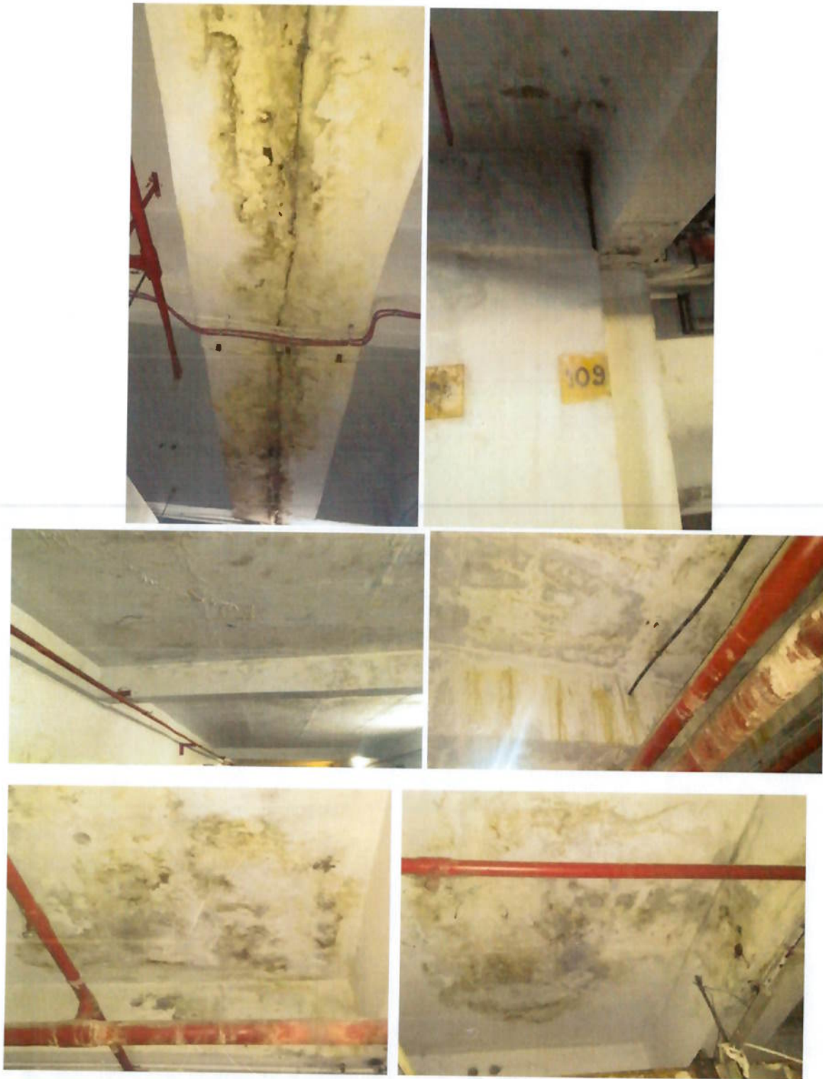
Fig. 6 Stains of water dampness/seepage on slabs and beams soffit
