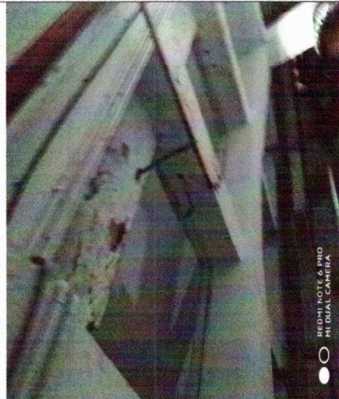
Leakages and peelings of paints on beams.
