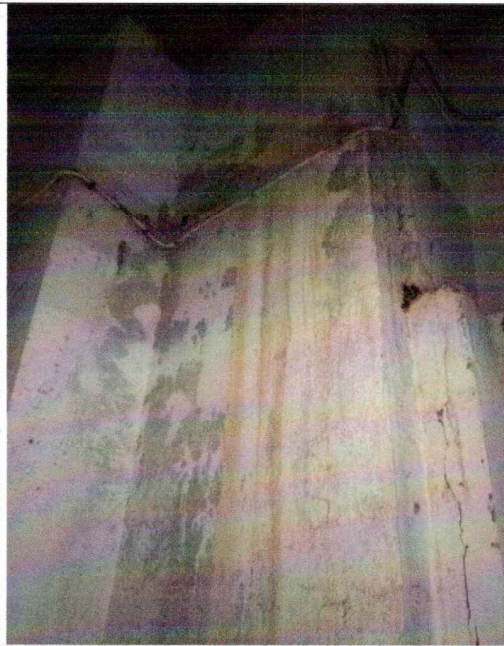
Leakages marks on column.
