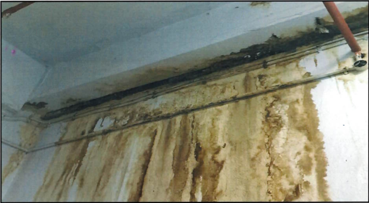
BAD CONDITION HAS BEEN NOTICED AT CONSTRUCTION JOINT
