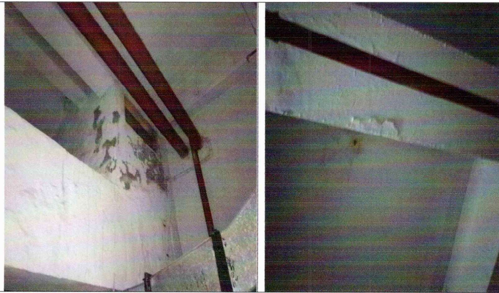
Dampness marks on column, beam.
