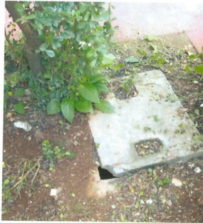
Fig. 11 Damaged Manhole covers
