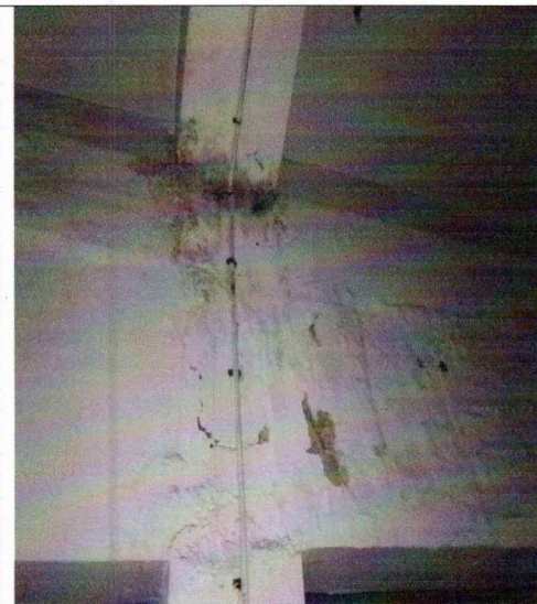
Peeling paints, bulging of plaster.
