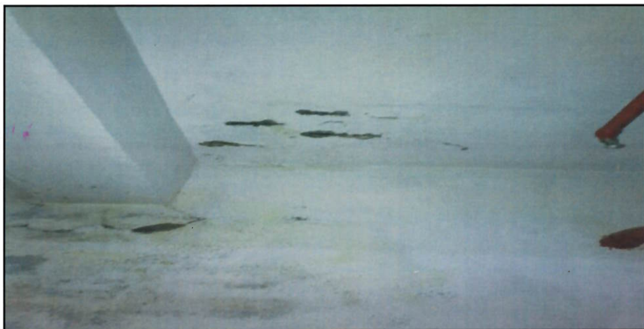
STEEL EXPOSED AT CEILING AREA
