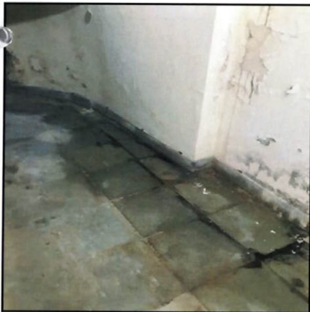
Joint Crack Heavy Leakage at Staircase area
