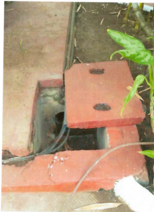
Fig. 12 Improperly closed drains
