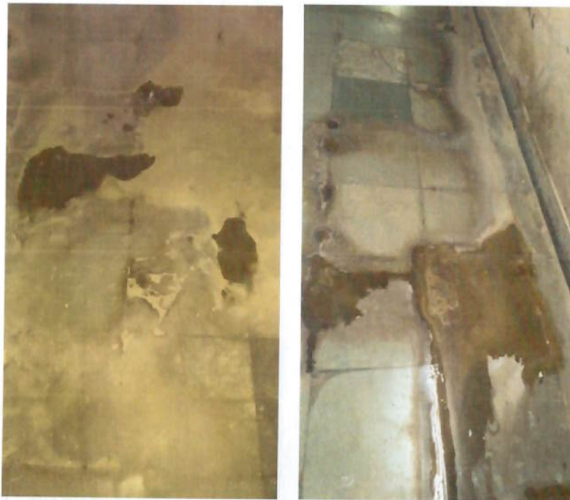
Fig. 2 Water oozing out from the gap between the floor tiles
