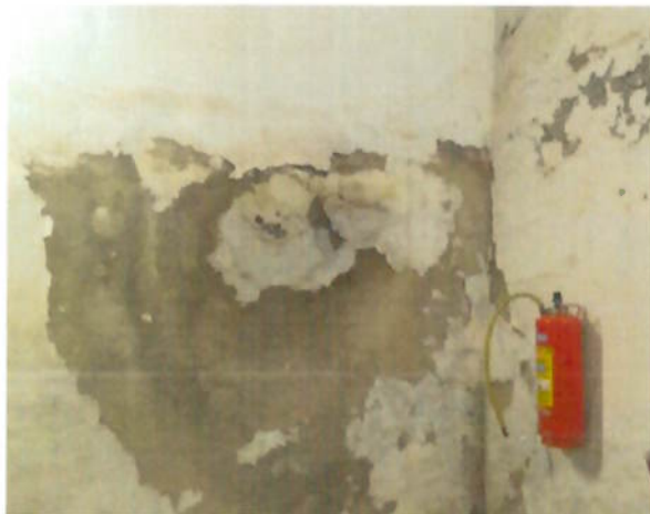
Fig. 3 Dry stains of dampness
