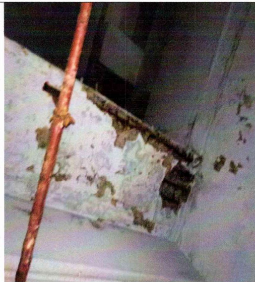
Spalled cover concrete with heavily exposed reinforcement at beam.
