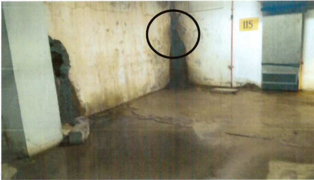
Fig. 4 Continuous water seepage from the wall
