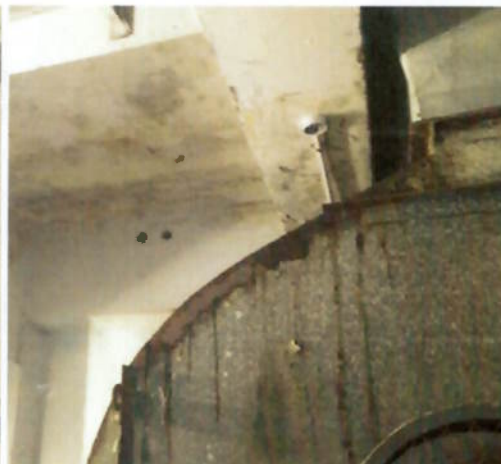
Fig. 3 Dry stains of dampness
