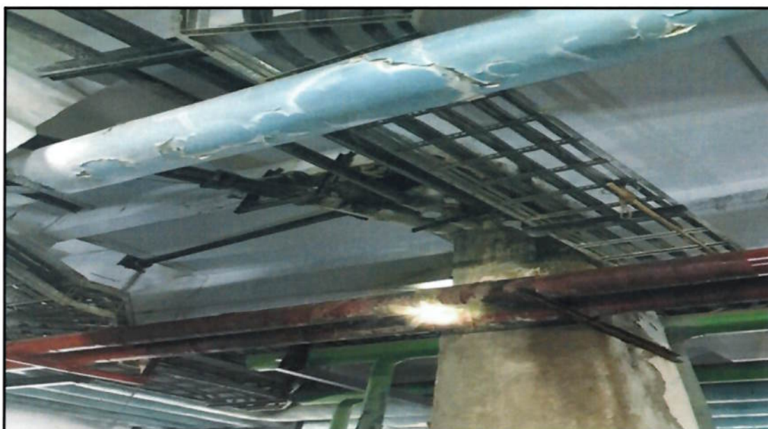
Heavy Leakage at Inlet and Outlet Pipes Beam Crack
