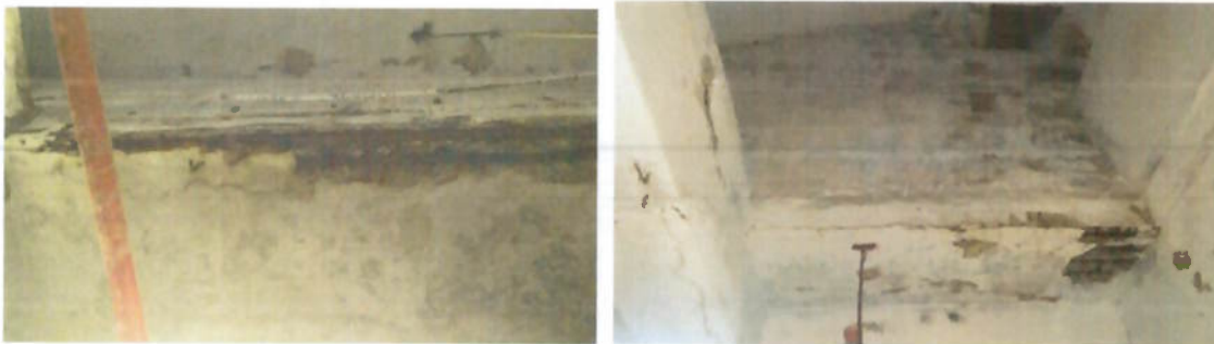
Fig. 8 Exposed corroded rods in beams
