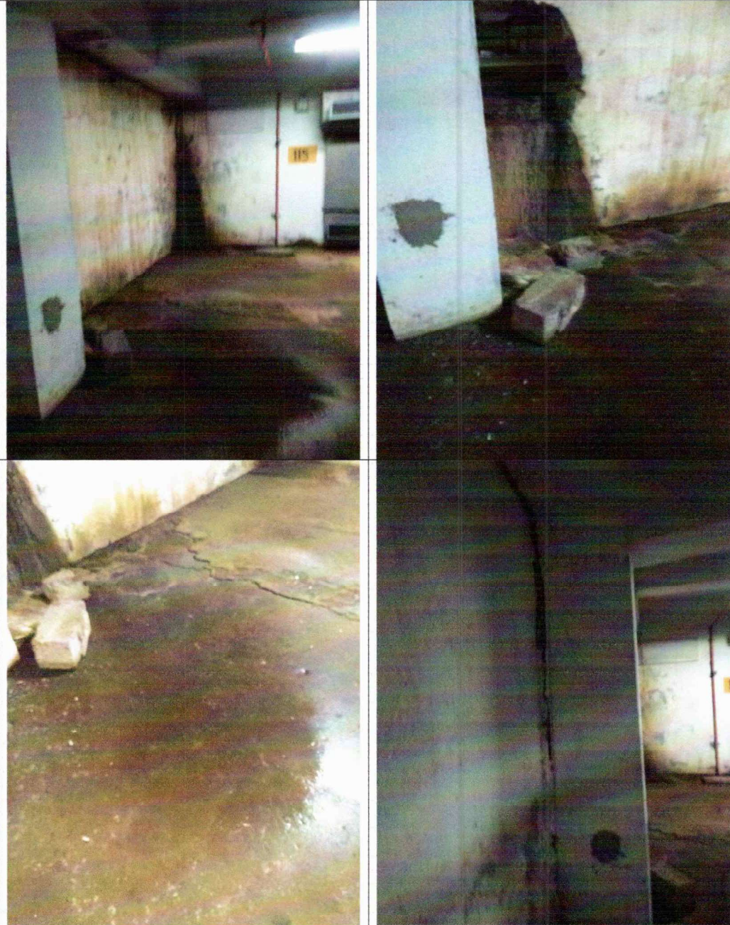
Leakages, exposed reinforcement at expansion joint beam, separation crack at column.
