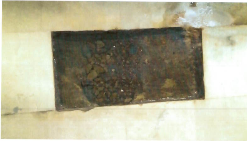
Fig. 1 Presence of water just below the tile at the basement
