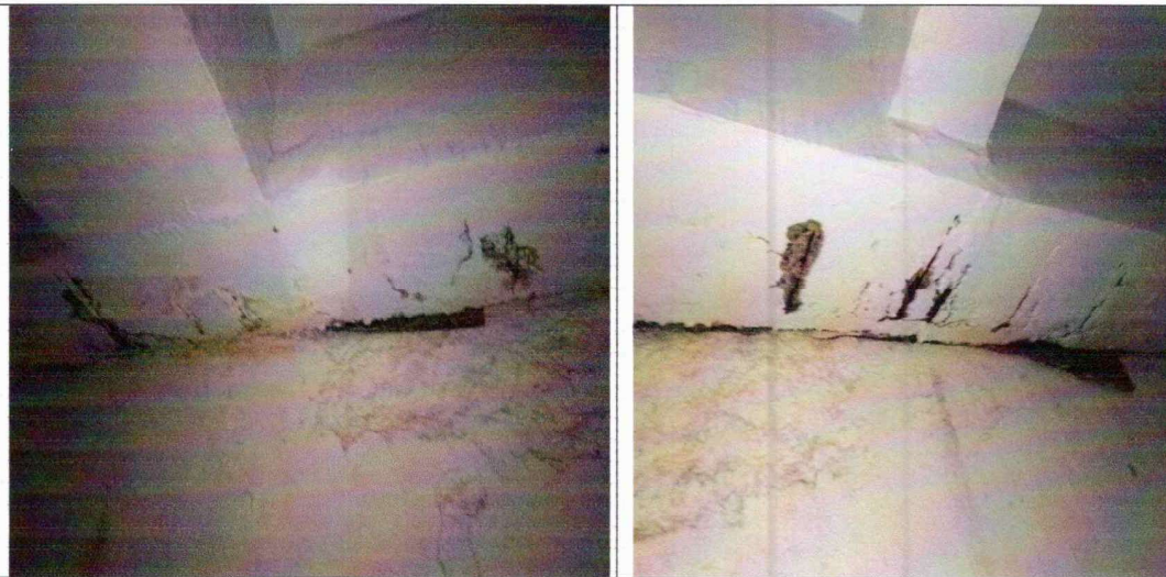
Spalled cover concrete with exposed reinforcement at beam.
