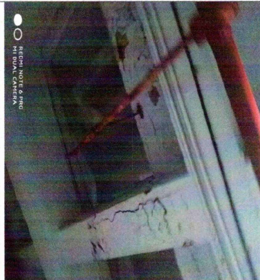
Cracks & bulging of plaster at beams.
