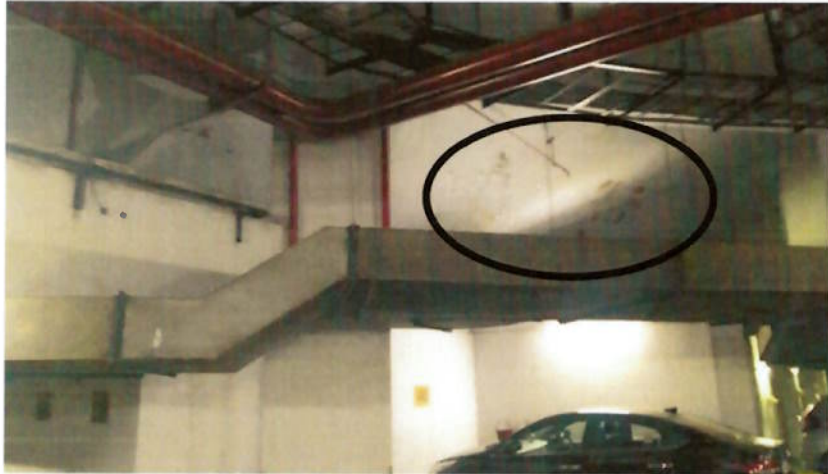
Fig. 7 Plaster peeling below the ramp (stairs)
